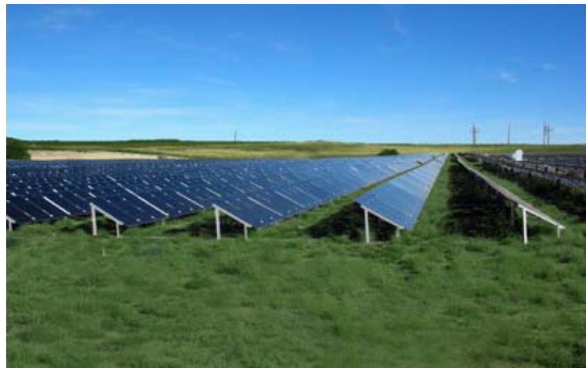
Photo courtesy of www.energy.gov.on.ca
